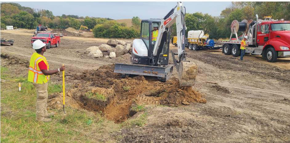
Installing fiber at a new build house jobsite near Kensington
