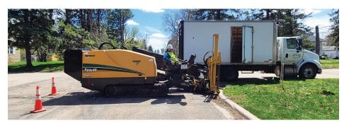
An Arvig Drill Operator runs the directional boring machine that allows the installation of fiber optic cable underground.
