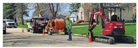
Runestone Telecom relies on contractors such as Arvig to do the construction of laying the main fiber optic cables. Once the main structures are buried, our crews work to run lines to residents and businesses for connection.
