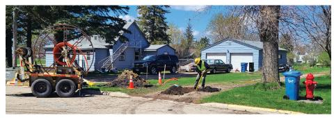
This crew worker is looking for buried facilities by making a series of small test holes, called "potholing." This is a method to accurately locate the underground lines.
